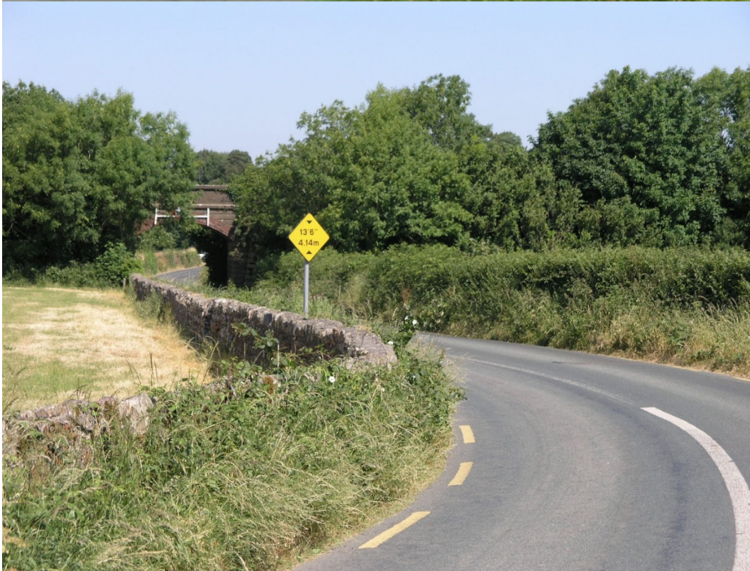
Figure 10.22: Dunbrody Bridge and Railway Bridge
