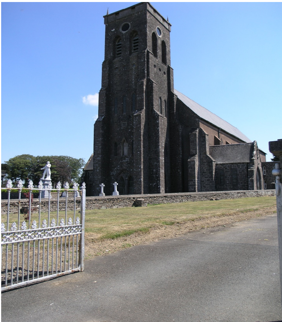
Figure 10.20: Pugin-designed church at Ramsgrange
